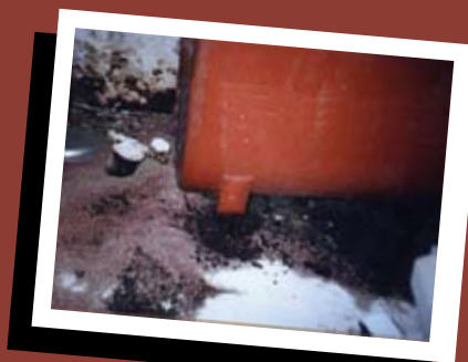
Corroded Leg
